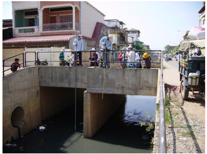
Figure 1 Sampling on the Trabek open interceptor sewer channel; an example of the underground pipe system discharging to the open channel can be seen lower left.
