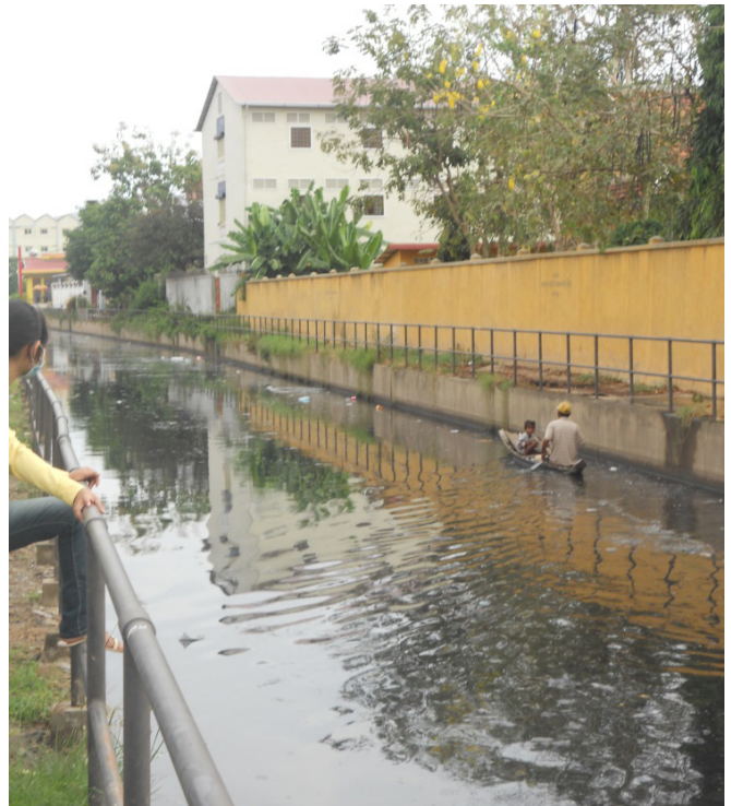
Figure 2 Trabek open interceptor sewer near the Trabek pump station.
